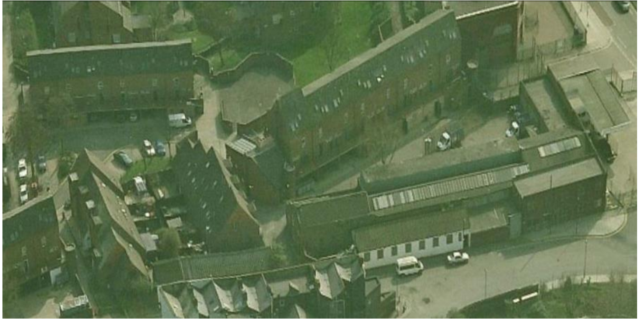
Image 1: Aerial view of the site viewed from the north
