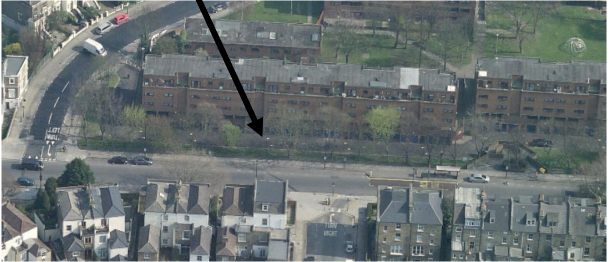
Image 1: Aerial Photo of the Front of the Site
